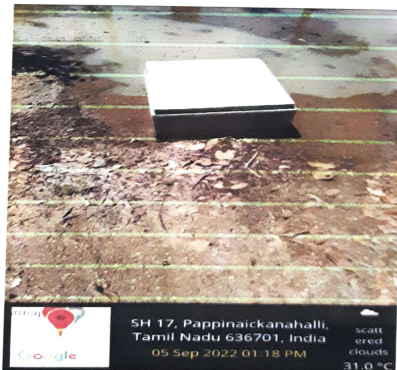
Waste Water Collection Point 2
