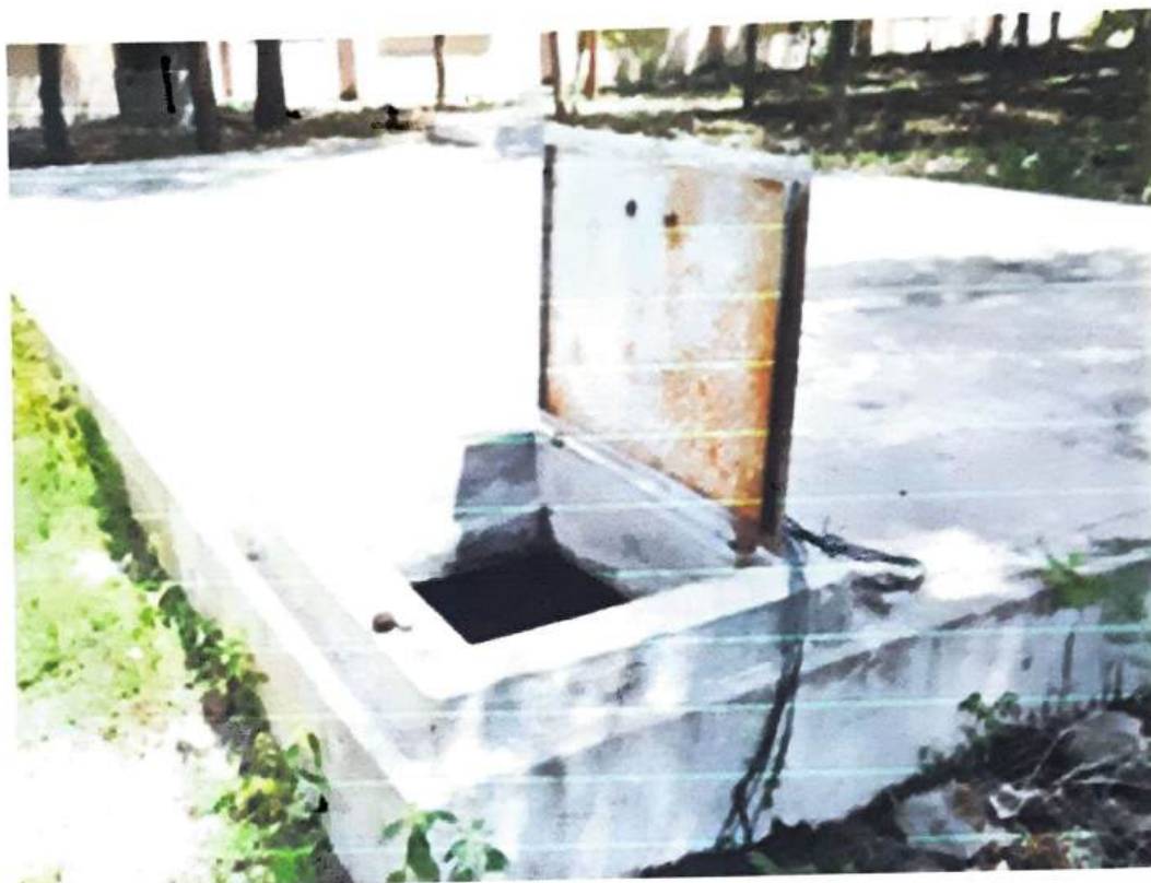
Rain Water Storage Tank (capacity - 50,000 liters)
