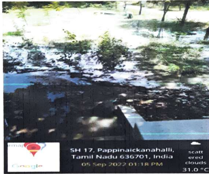
Rain Water Collection Junction
